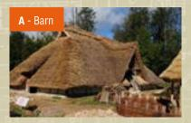
The barn is the largest building at Campus Galli to date. The floor area measures approx.  $11 \times 21.8$  m, the height approx. 8 m. The roof is covered with local rye straw.
